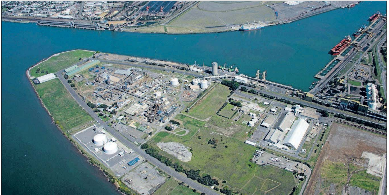
POTENTIAL: The Walsh Point precinct is one of the three sites for additional fuel storage within the Port of Newcastle. Image: Port of Newcastle
